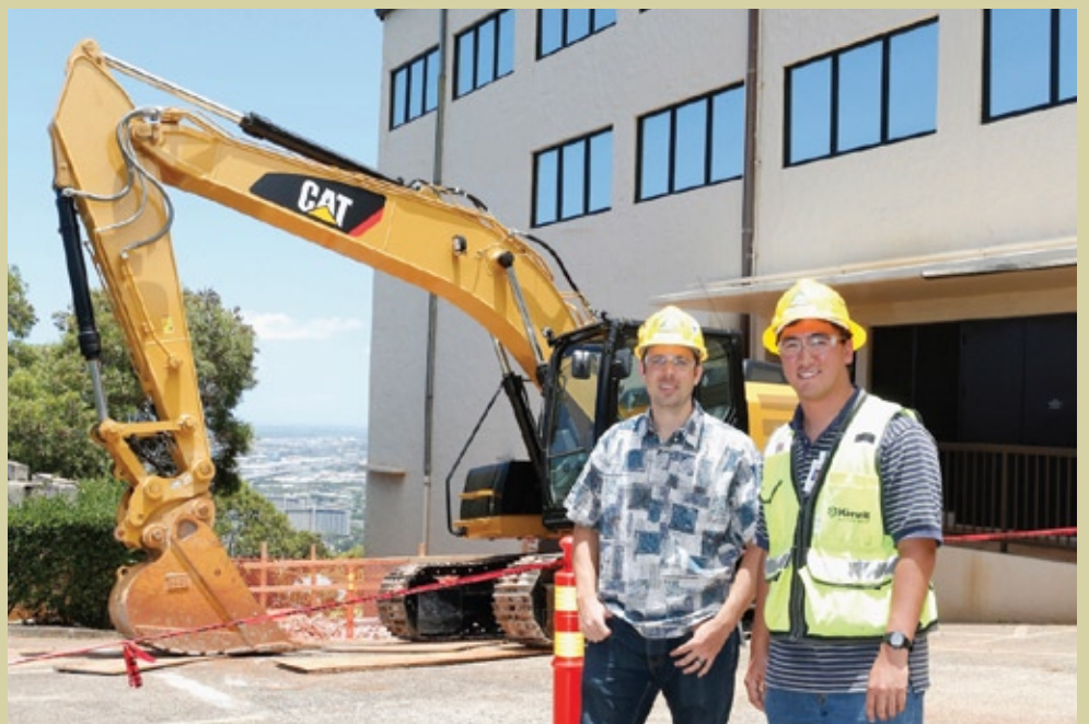
Special projects manager, Jesse Dowsett KSK'02, and engineering intern, Christian Brown KSK'10, of the Kiewitt Building Group at a KS Kapālama construction site near 'Akahi dining hall.
